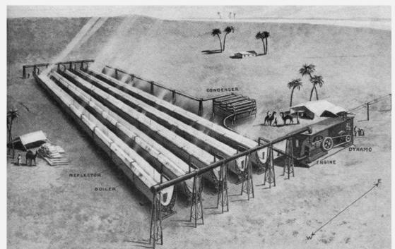
Figure 1: Concentrated solar power plant in Maadi (Egypt), built in1897(RAGHEB, 2011)
